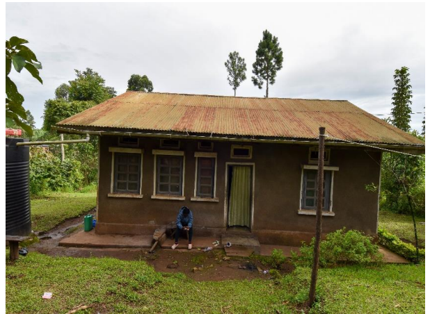
Sector office at Ndekye to be renovated
