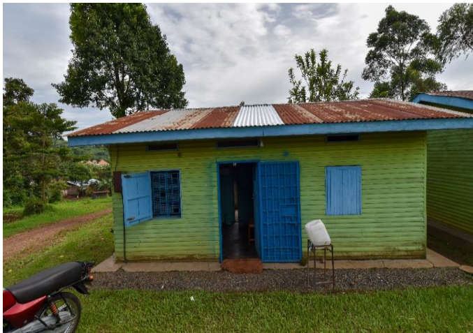
Staff house at Ndekye to be renovated
