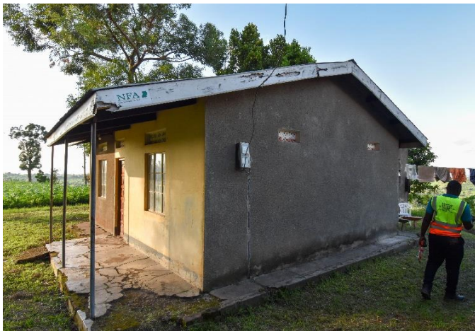
Consulting Team carrying out dilapidation analysis at Katerera
