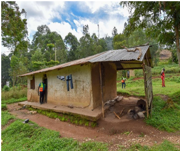
Staff house at Bihanga station
