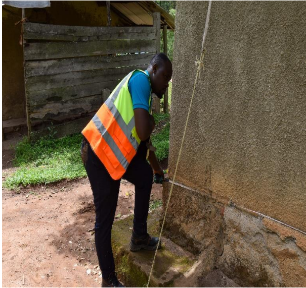
Consulting team taking measurements at Bihanga Station
